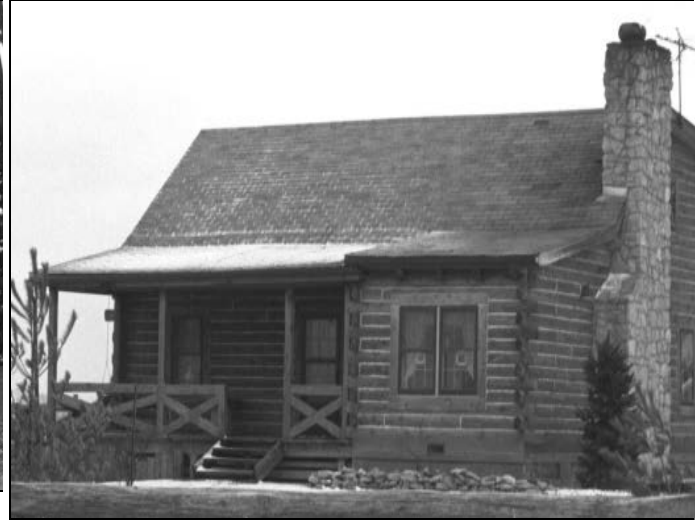
Grade C Log Home Residential Dwelling
