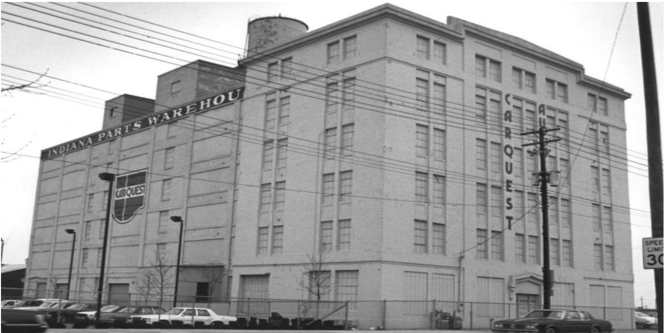
Grade C Loft Warehouse
