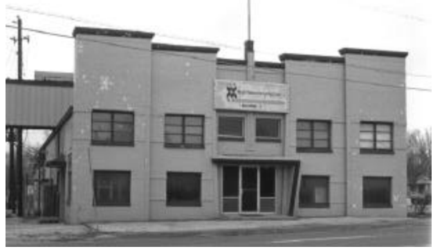
Grade C Industrial Facility
