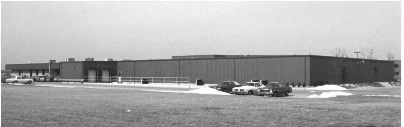
Grade C Light Industrial Facility
