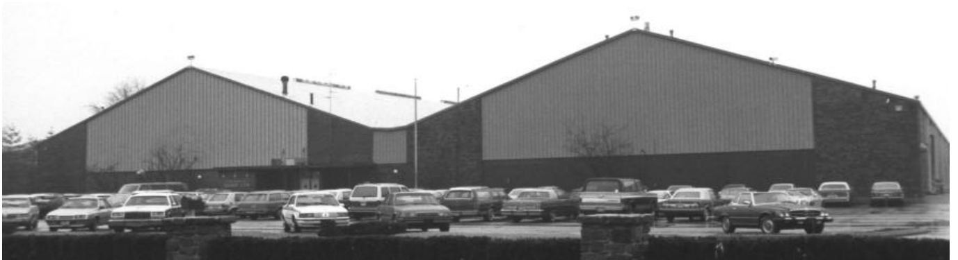
Grade C Light Warehouse
