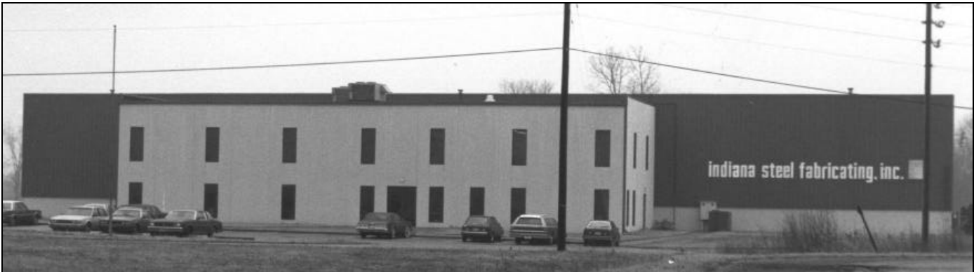
Grade C Industrial Facility
