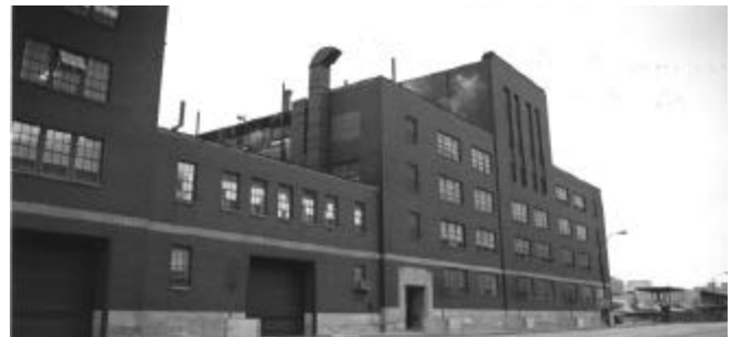
Grade C Loft Factory
