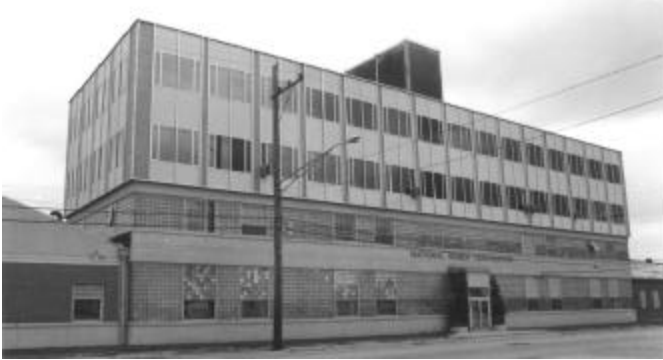
Grade C Industrial Office
