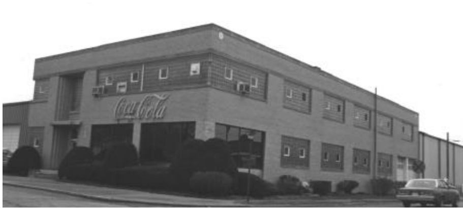
Grade C Industrial Facility
