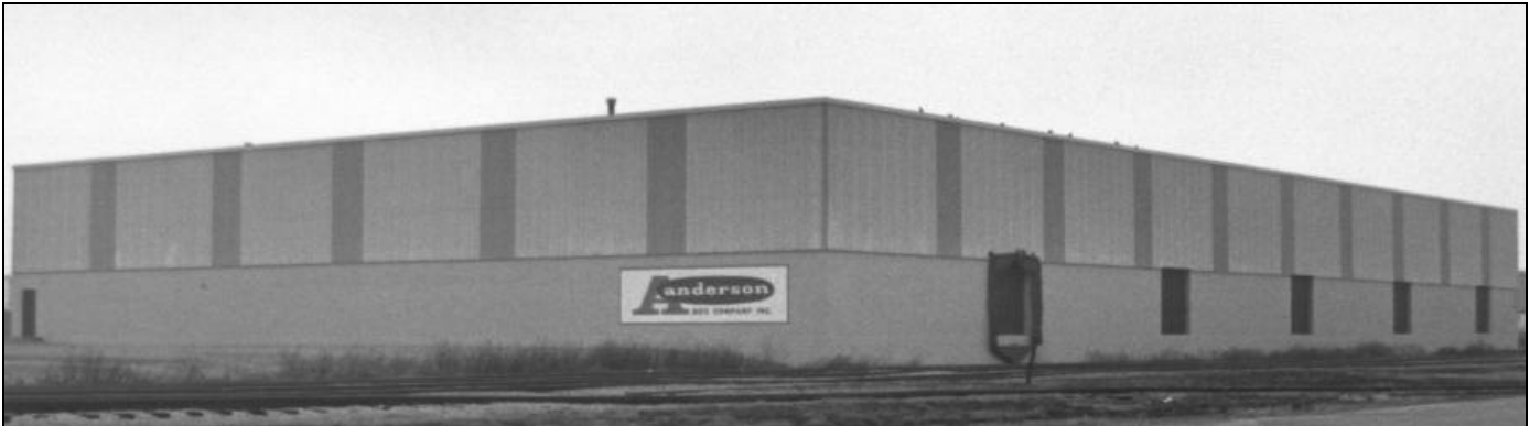
Grade C Light Warehouse
