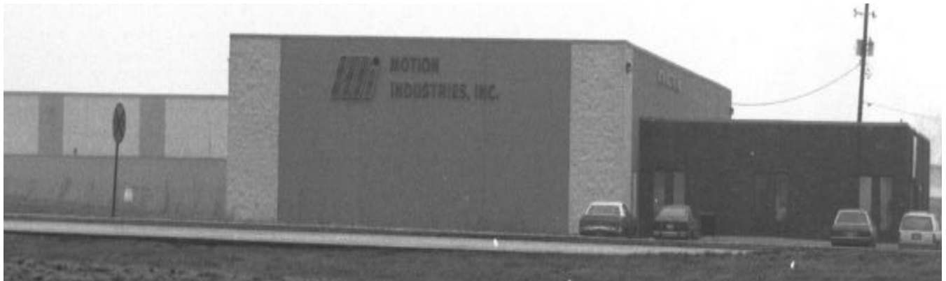
Grade C Light Industrial Facility
