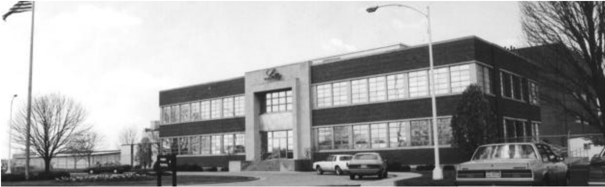
Grade B Industrial Office
