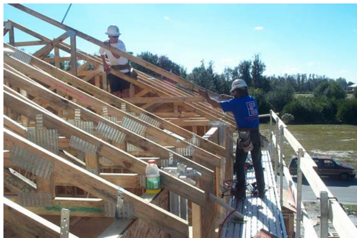
Figure 2 - Workers using an exterior bracket scaffold to install roof trusses.
