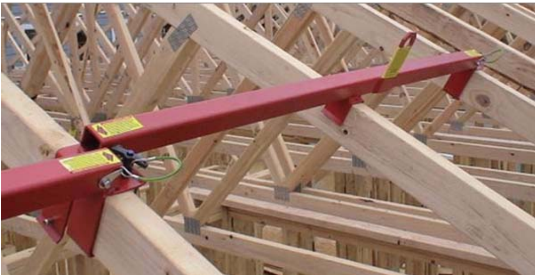
Figure 4 – An example of a spreader attached to roof trusses.
