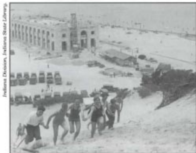
View of the nearly completed Pavilion at the Indiana Dunes State Park, circa 1930.
