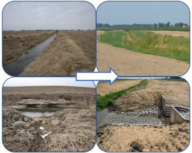
Before (left) and after (right) showing BMP implementation on Stump Ditch. The two-stage ditch increases bank stability while improving drainage and ecological functions. Photos courtesy of Clinton County SWCD.
