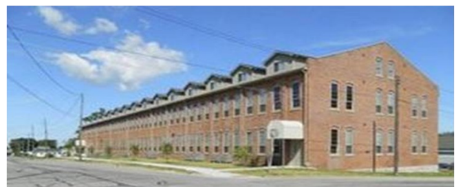
Former Bromwell Brush & Wire Goods Company, Greensburg: After (August 2015)
