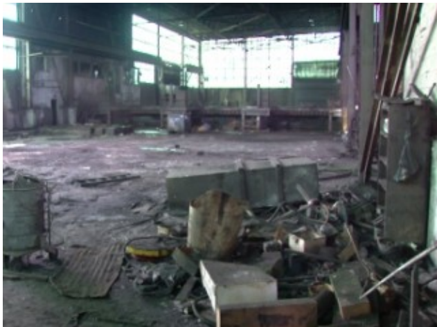
Former Elkhart Foundry—Before Demolition
