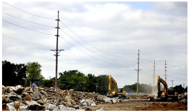
Former Elkhart Foundry—After Demolition
