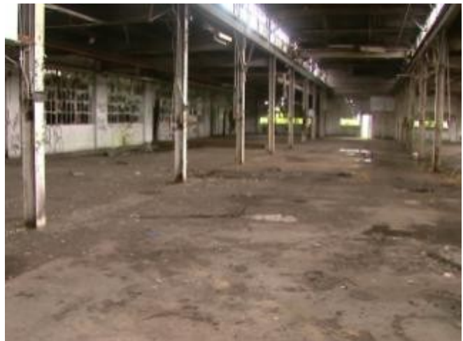
Former LaBour Pump—Before Demolition
