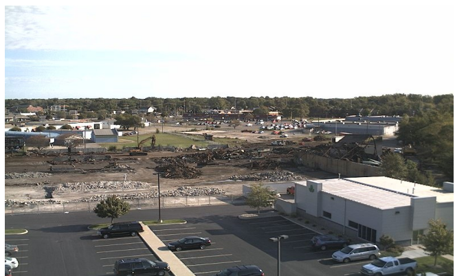
Former LaBour Pump—During Demolition
