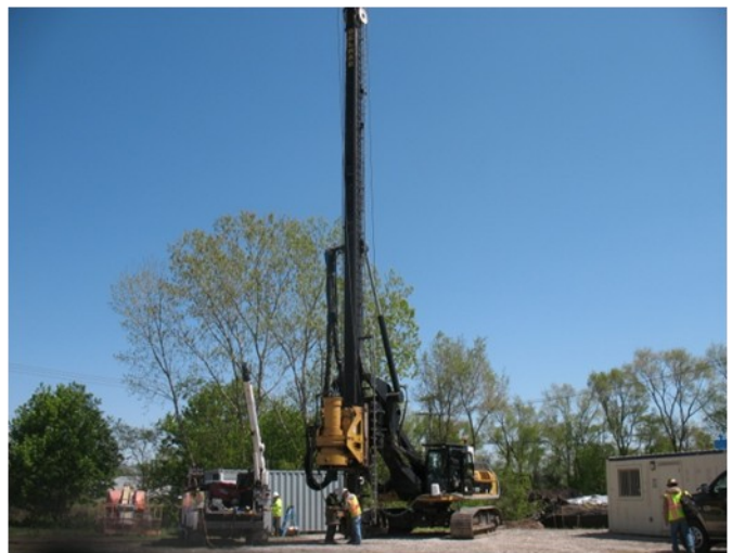
Former Columbus Wood Treating Plant – during remediation
