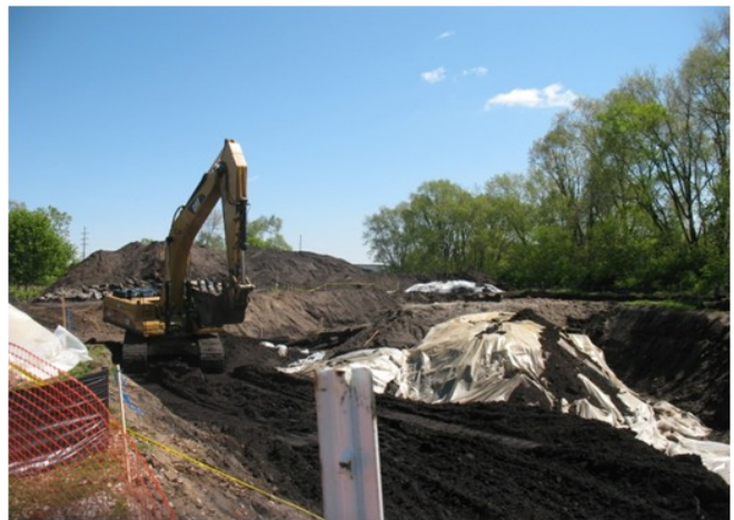
Former Columbus Wood Treating Plant – during remediation
