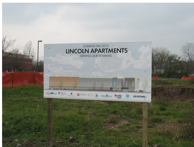
Before: Former National Malleable Castings Company, 2732 W Michigan Street/530 N. Holmes Avenue
