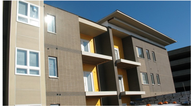
After: Illinois Place Apartments
