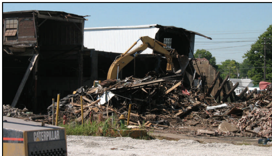
The former Ertel Manufacturing buildings were demolished in August 2007.
