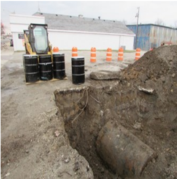
Southside Lumber, Kokomo – UST removal
