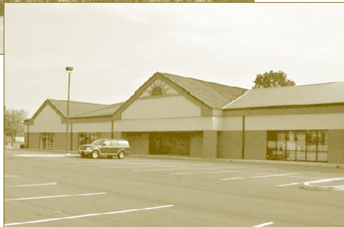
A former Lincoln Avenue gas station is now a retail shop.
