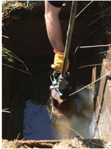
Figure 17.17.1 Enigma-hyQ logger installed on 500 mm PVC main via fire hydrant. (Source: Primayer)
