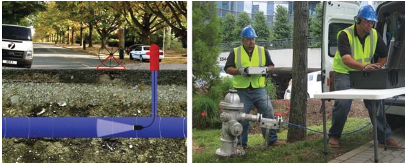
Figure 5.2 Push tethered system which can be operated with or against the water flow with access through tapping point or fire hydrant. (Source: JD7 Ltd)
