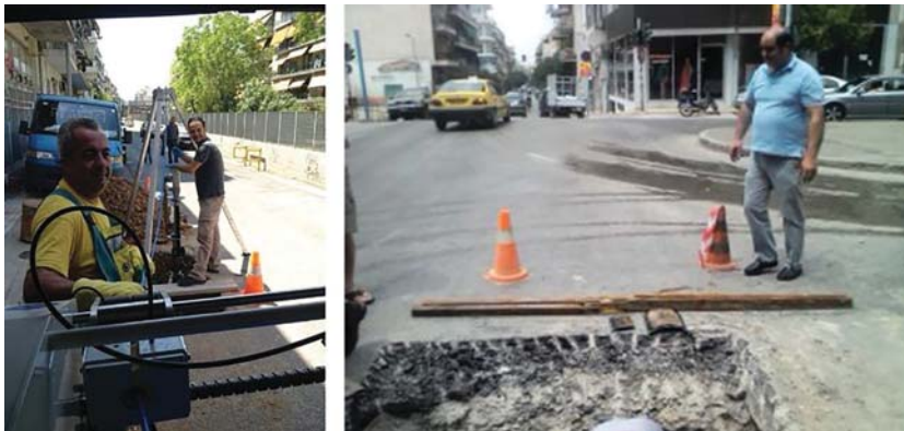
Figure 17.7.1 Team operating JD7 LDS1000 in Greece. (Source: JD7 Ltd)
