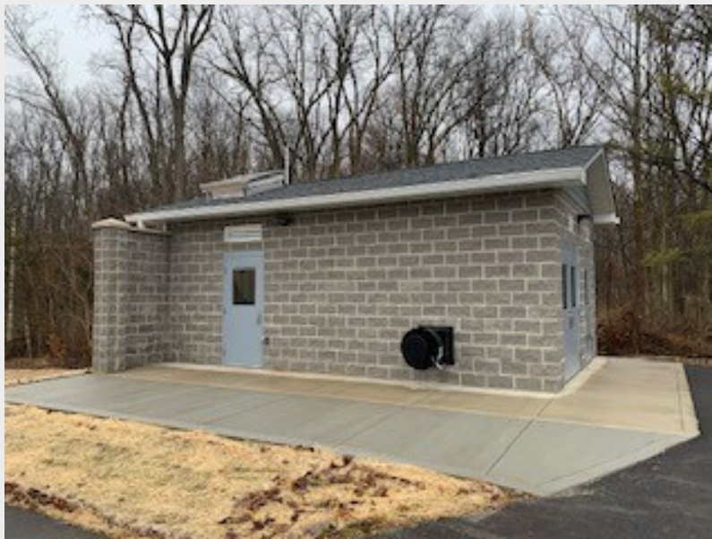
Above: New Well House in Delphi, Indiana funded through the Indiana State Revolving Fund (SRF).
