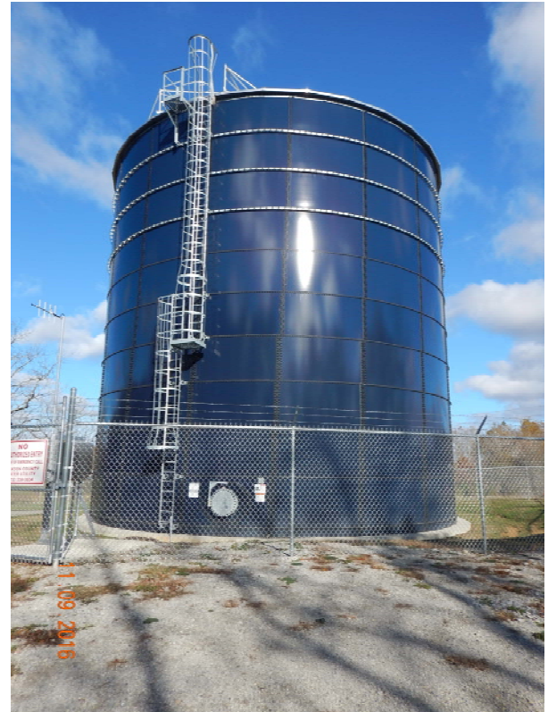
Jackson County Water Utility: New 600,000 Gallon Water Storage Tank
