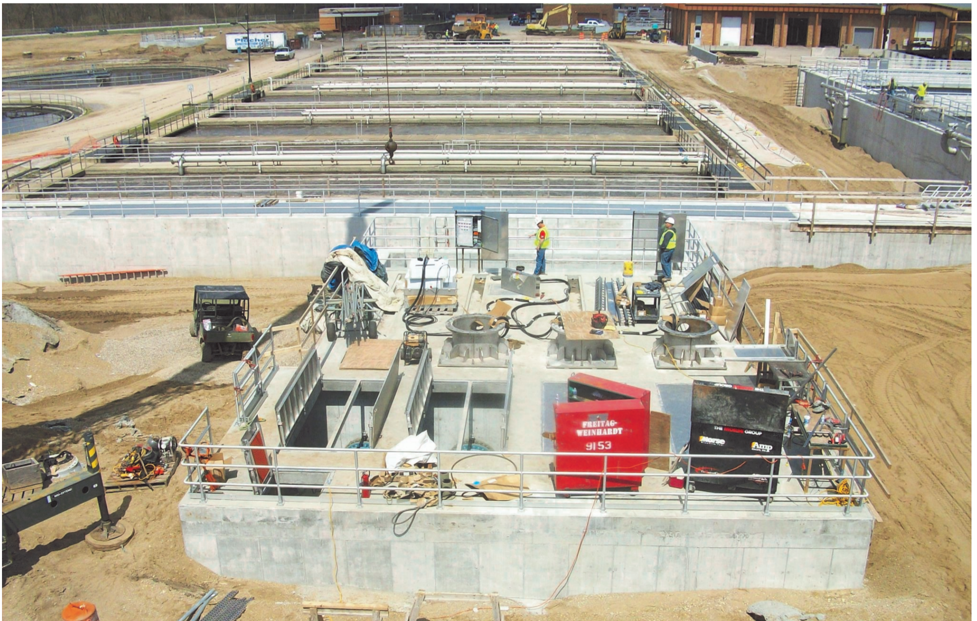
Installation of Terre Haute's Recycle Pump Station
