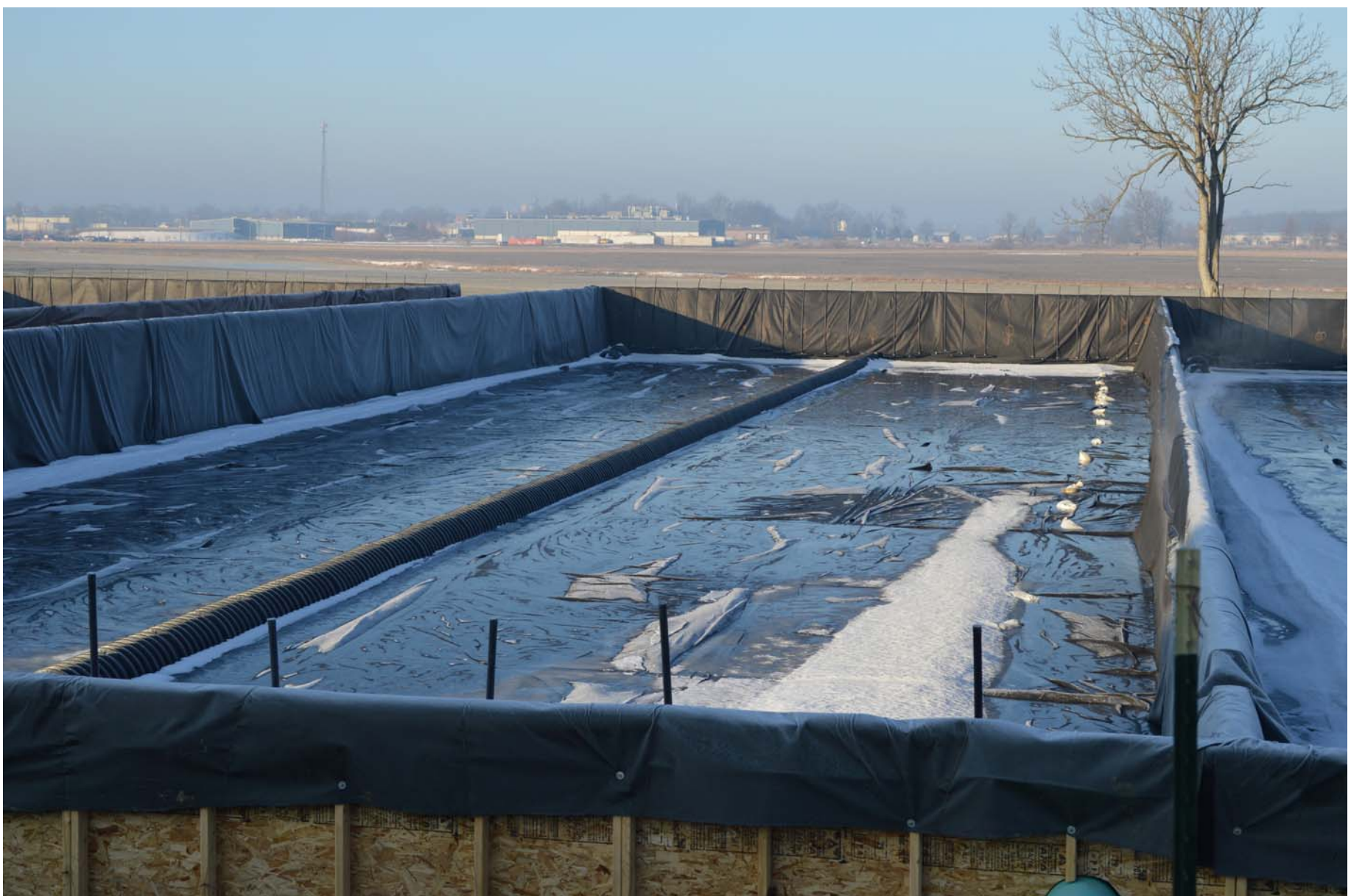
Berne's Submerged Attached Growth Reactor (SAGR) cells under construction.
