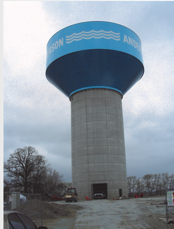
New 2.0 million gallon elevated water storage tank to provide safe drinking water to the city.
