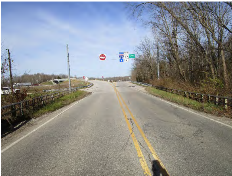
PHOTO 9: LOOKING AT NORTH APPROACH FROM END OF BRIDGE
