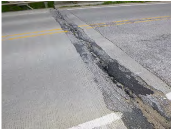
SOUTH BRIDGE JOINT
