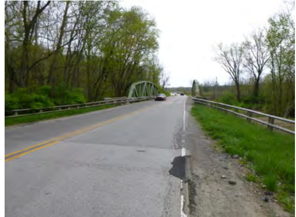
APPROACH LOOKING SOUTH
