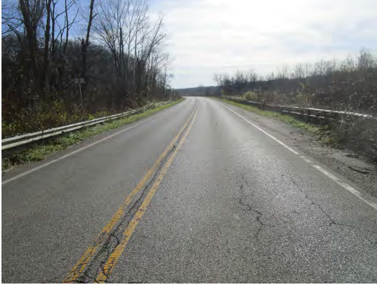
PHOTO 10: LOOKING AT SOUTH APPROACH FROM END OF BRIDGE
