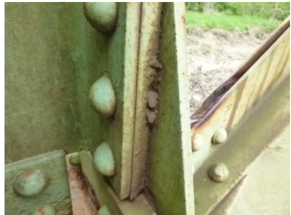
TACK WELD SOUTHWEST L3
