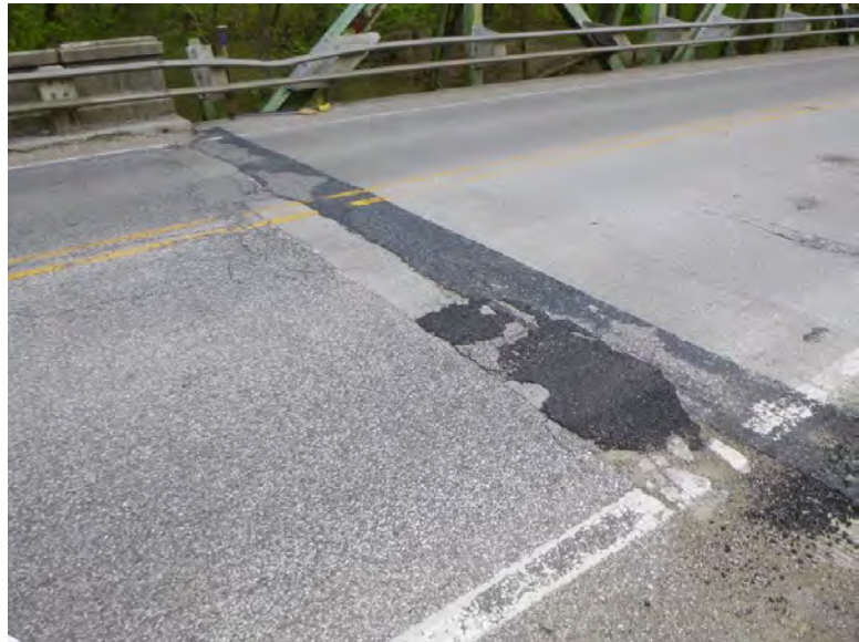
PHOTO 20: NORTH BRIDGE JOINT
