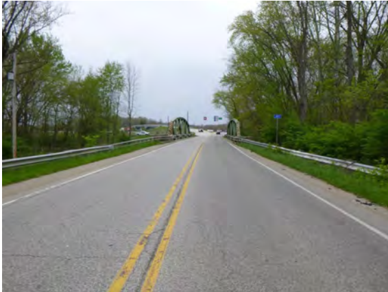
APPROACH LOOKING NORTH
