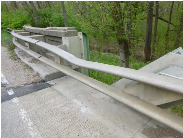
PHOTO 24: SOUTH BRIDGE JOINT
