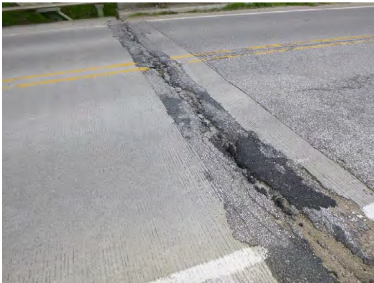
PHOTO 21: SOUTH BRIDGE JOINT
