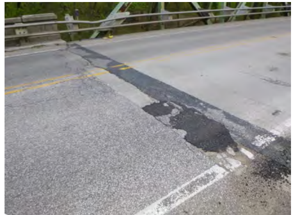
NORTH BRIDGE JOINT
