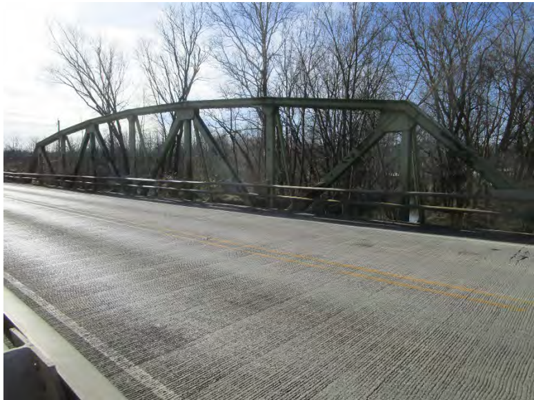
PHOTO 5: WEST TRUSS LOOKING FROM DECK
