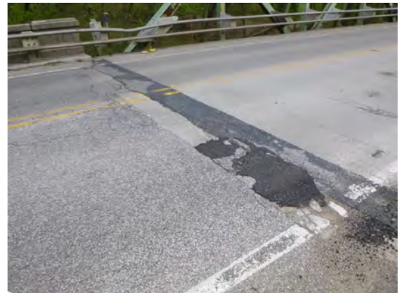
NORTH BRIDGE JOINT
