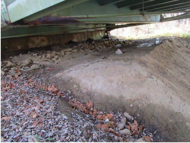
PHOTO 4: TYPICAL FLOOR SYSTEM
