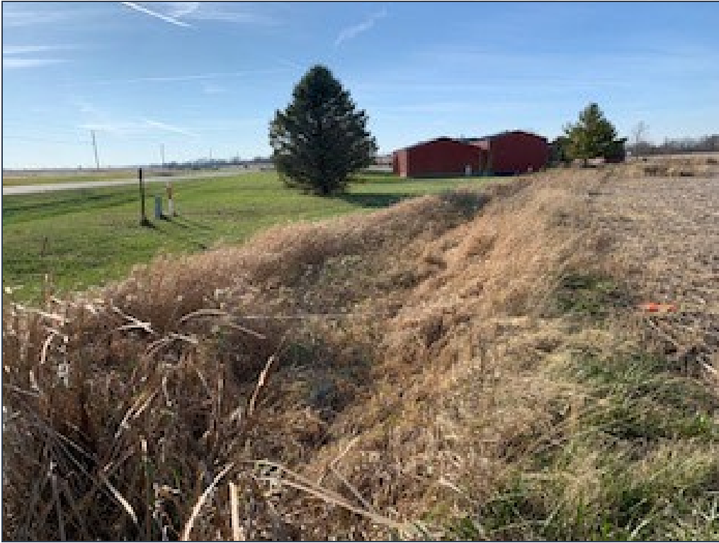
Dry Grass Swale, Hendricks County, Indiana
