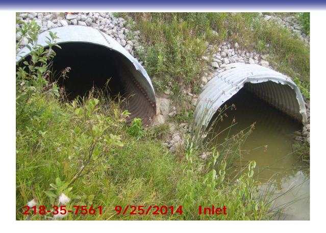
Double culverts with one set higher to avoid sediment accumulation.
