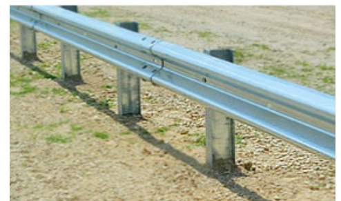
Figure 11-2 MGS W-Beam Midspan
