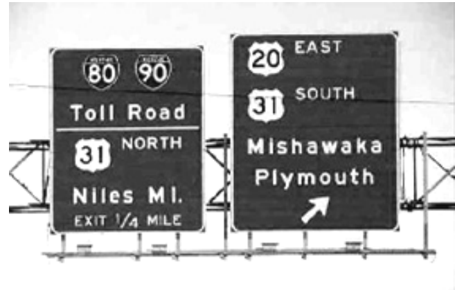
Figure 3-1 Overhead Sign Structure
