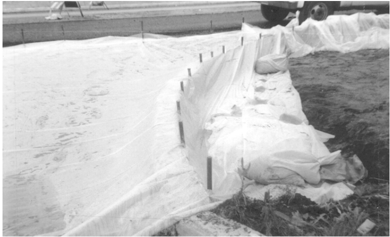
Figure 7-4 Curing with Plastic Sheeting
