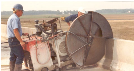
Figure 9-4 Sawing Concrete Joint
