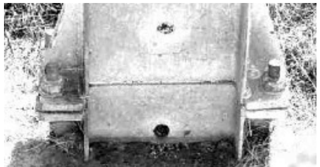
Figure 2-4 Structural Steel Post on a Breakaway Stud
