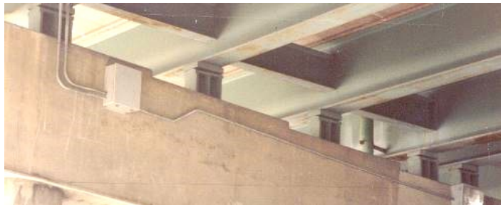
Figure 4-3 Acceptable Underpass Circuitry
