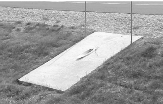
Figure 10-5 Underdrain Outlet Protector
