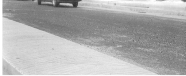
Figure 5-2 Concrete Center Curb
