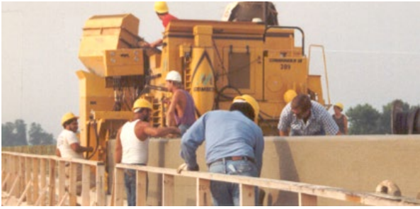
Figure 9-2 Hand-finishing Concrete Barrier
