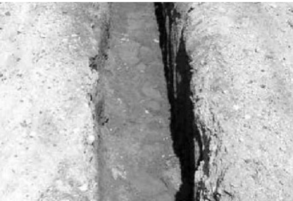
Figure 10-3 Underdrain Trench
