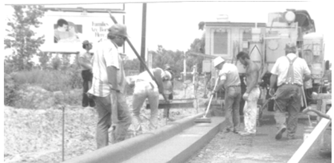
Figure 5-1 Combined Curb and Gutter
