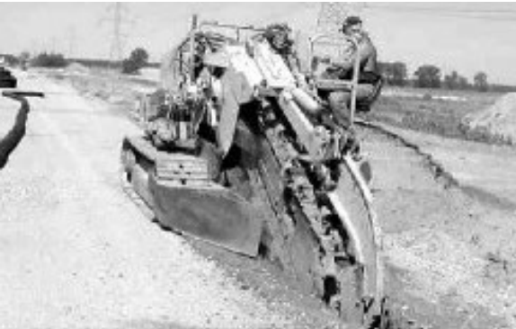
Figure 10-2 Underdrain Trencher
