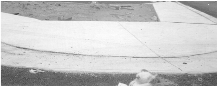
Figure 6-2 Contraction and Preformed Joints
