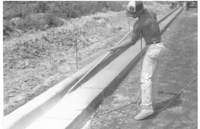
Figure 5-5 Applying Curing Compound
