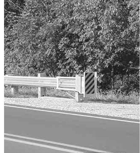
Figure 11-4 Guardrail End Treatment
