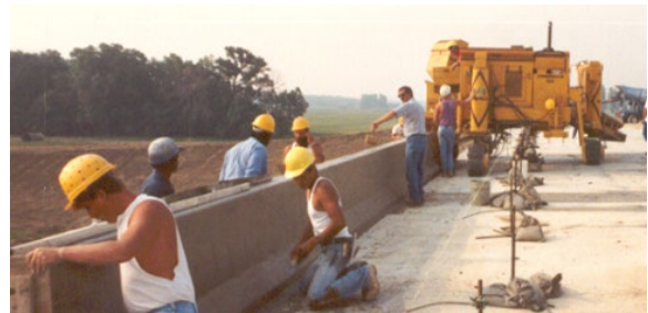
Figure 9-1 Slip-forming a Concrete Barrier
