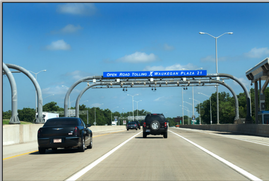
Figure 2-3: Monotube Toll Gantries (Illinois Tollway)
