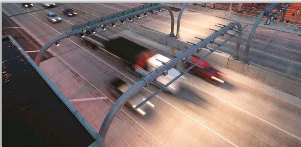
Figure 2-1: Example of an AET System Toll Zone
