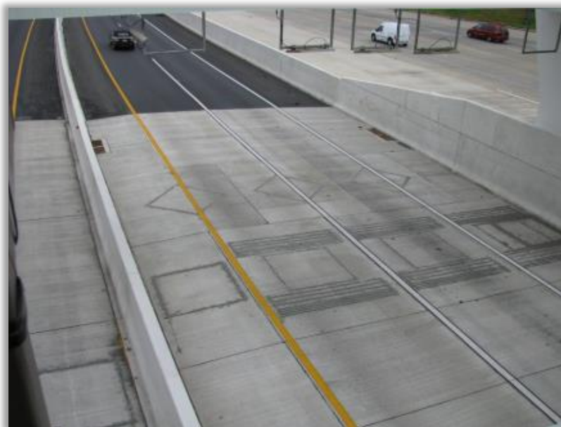
Figure 2-7: Example of Axle-Based AVDC Loop Layout Installation
