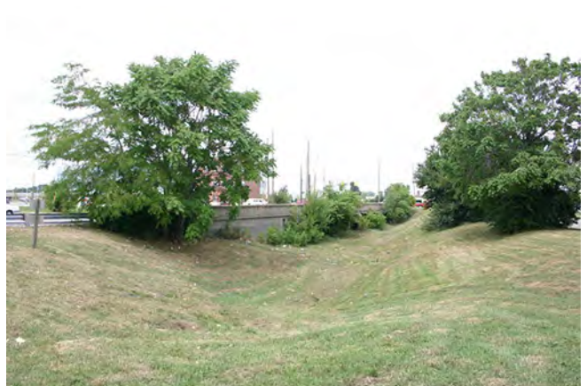
6_Looking NW at the SE section of Bridge 2410F
