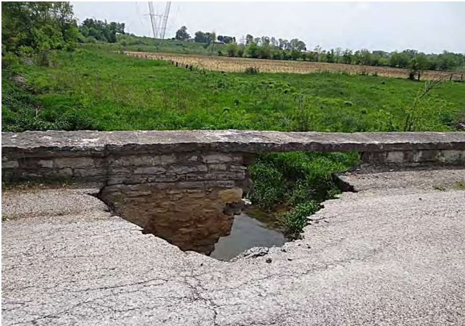
05/16/2013 Shelby County Bridge 149 photos The hole continues to grow as the arch continues to deteriorate. Shelby County has placed riprap and "No Trespassing" signs to deter the public. Attachment 24
