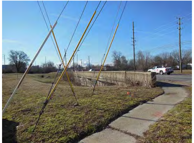
4_Bridge 2410F E elevation looking SW
