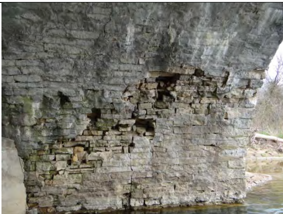
Figure 2 - Pier 2, east face - 2012
