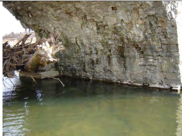
Figure 5 - West Face of Pier 3 - 2006
