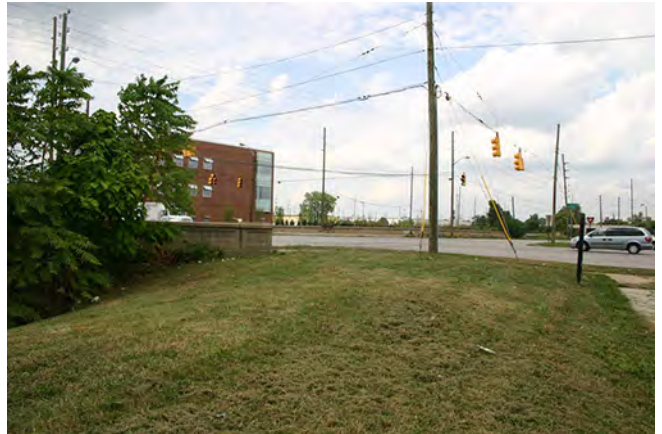
4_Looking NW at Bridge 2410F from the SE quadrant of the intersection
