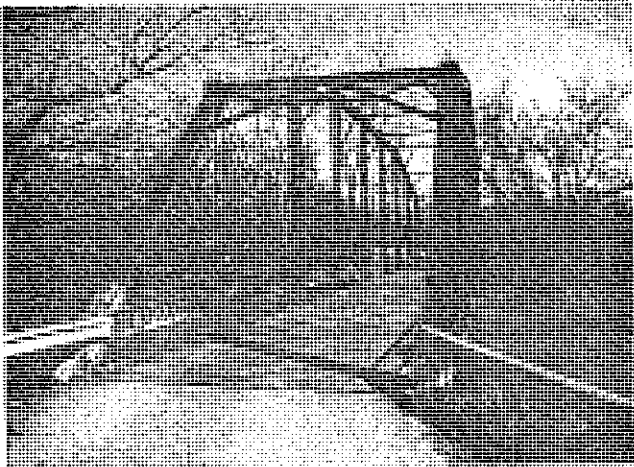
View north along CR 800 East
