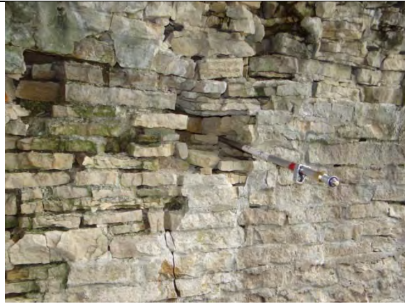
Figure 3 - 2012 - Looking at Pier 3 west face - note probe
