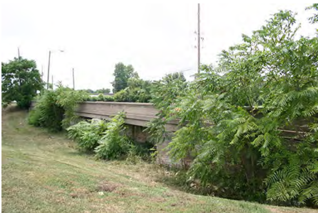
5_Looking SW from the SE quadrant of the intersection
