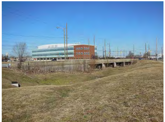
6_Bridge 2410F E elevation looking NW
