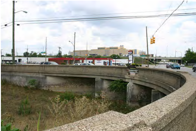
3_Looking E at the NW section of Bridge 2410F
