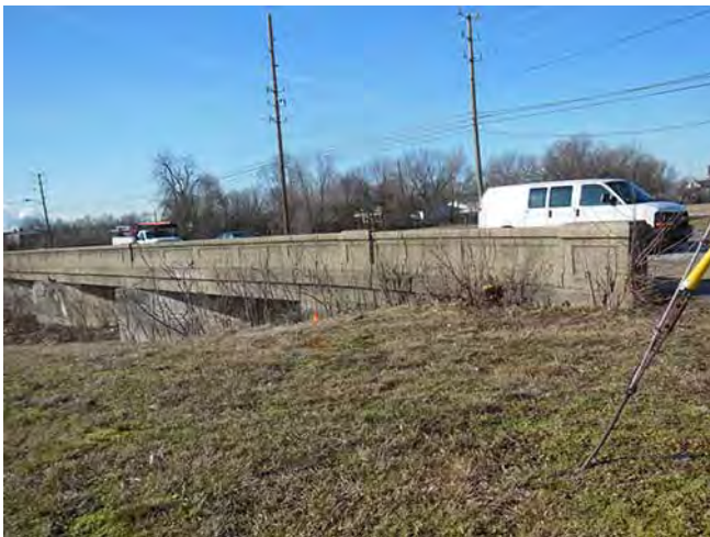
5_Bridge 2410F E elevation looking SW
