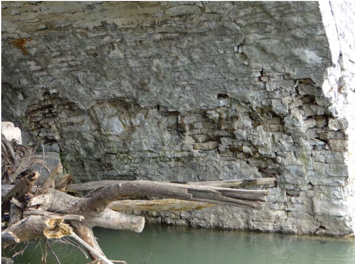
Figure 1 - West Face of Pier 3 - 2012.
