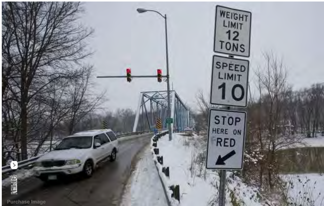
A car comes over the Indiana 225 bridge near Battle Ground. The Indiana Department of Transportation has placed a 12-ton weight limit and 10 mph speed limit on the bridge that spans the Wabash River in Tippecanoe County. / Michael Heinz/Journal & Courier
