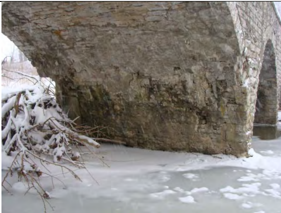
Figure 4 - West Face Pier 3 - 2009
