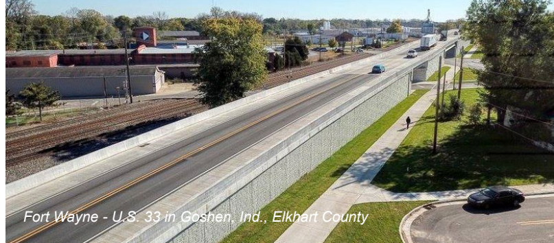
Crawfordsville - I-65 Major Moves, Tippecanoe County
