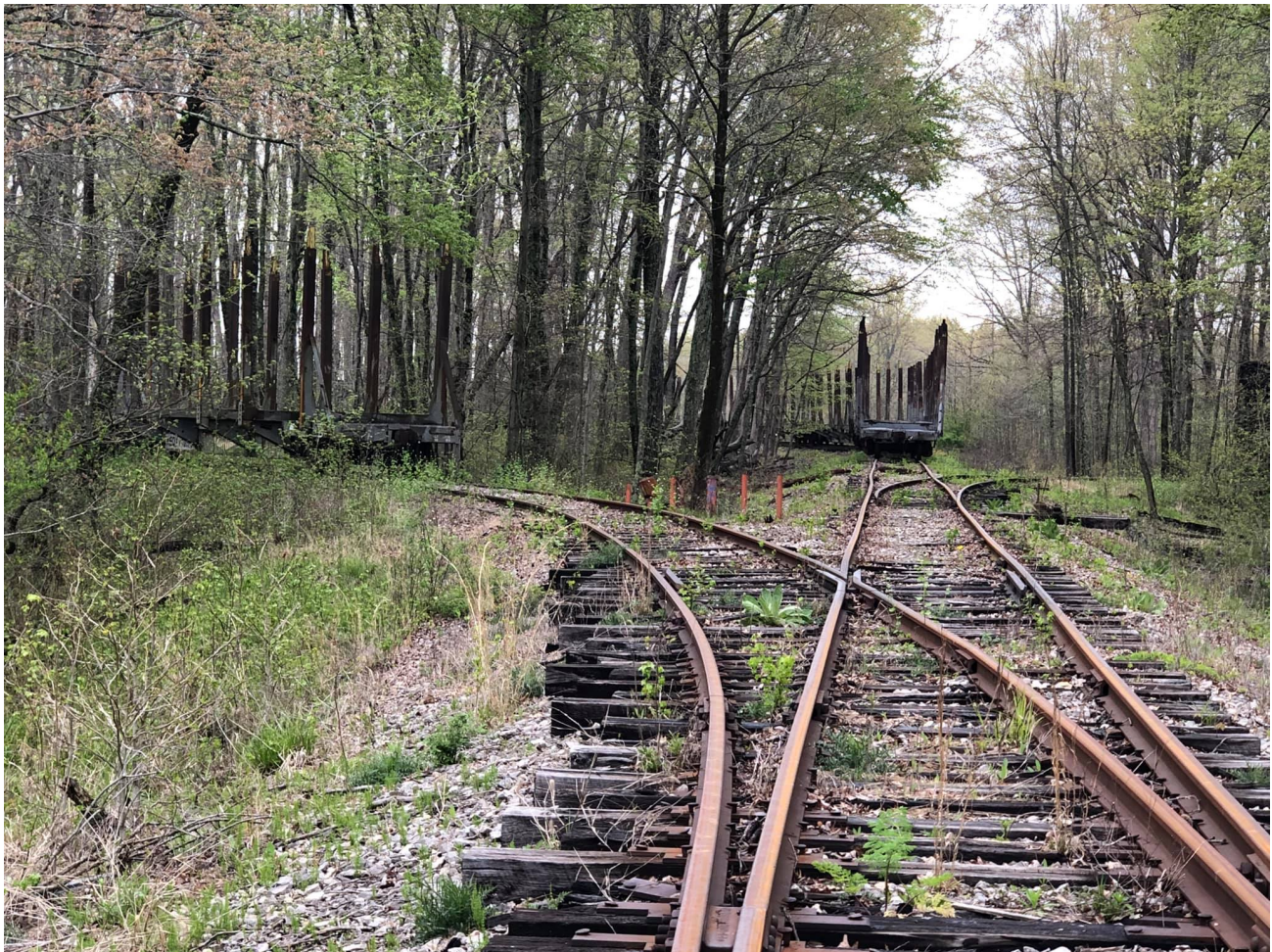
Figure 2-11 – Abandoned Rail Infrastructure at Jefferson Proving Grounds
