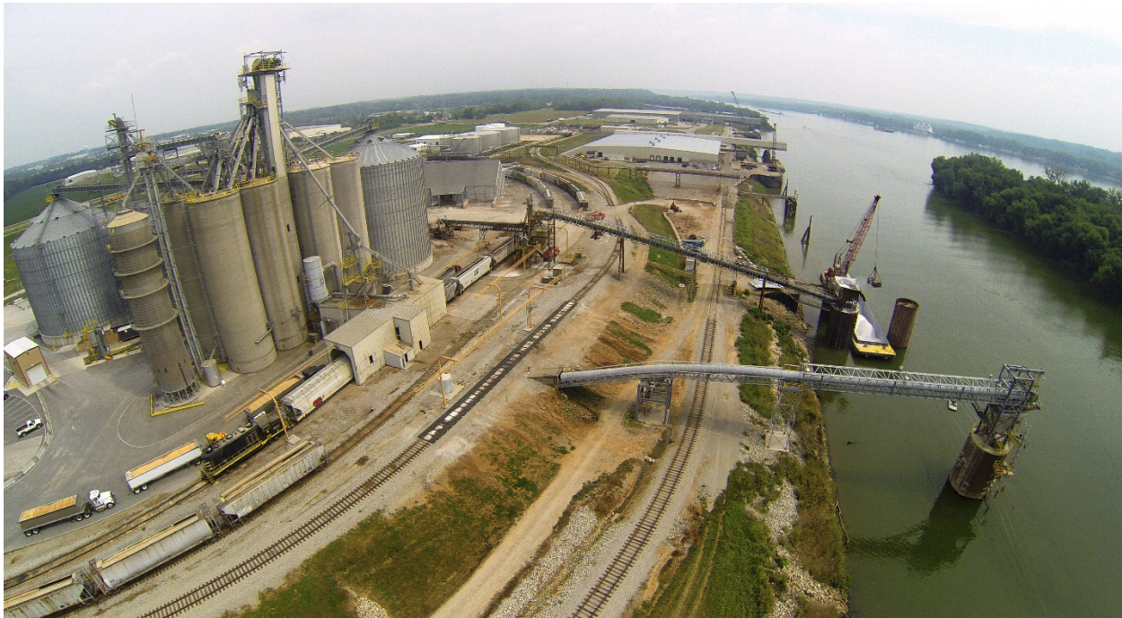
Figure 2-17 – Rail Infrastructure between Consolidated Grain & Barge and the Ohio River
