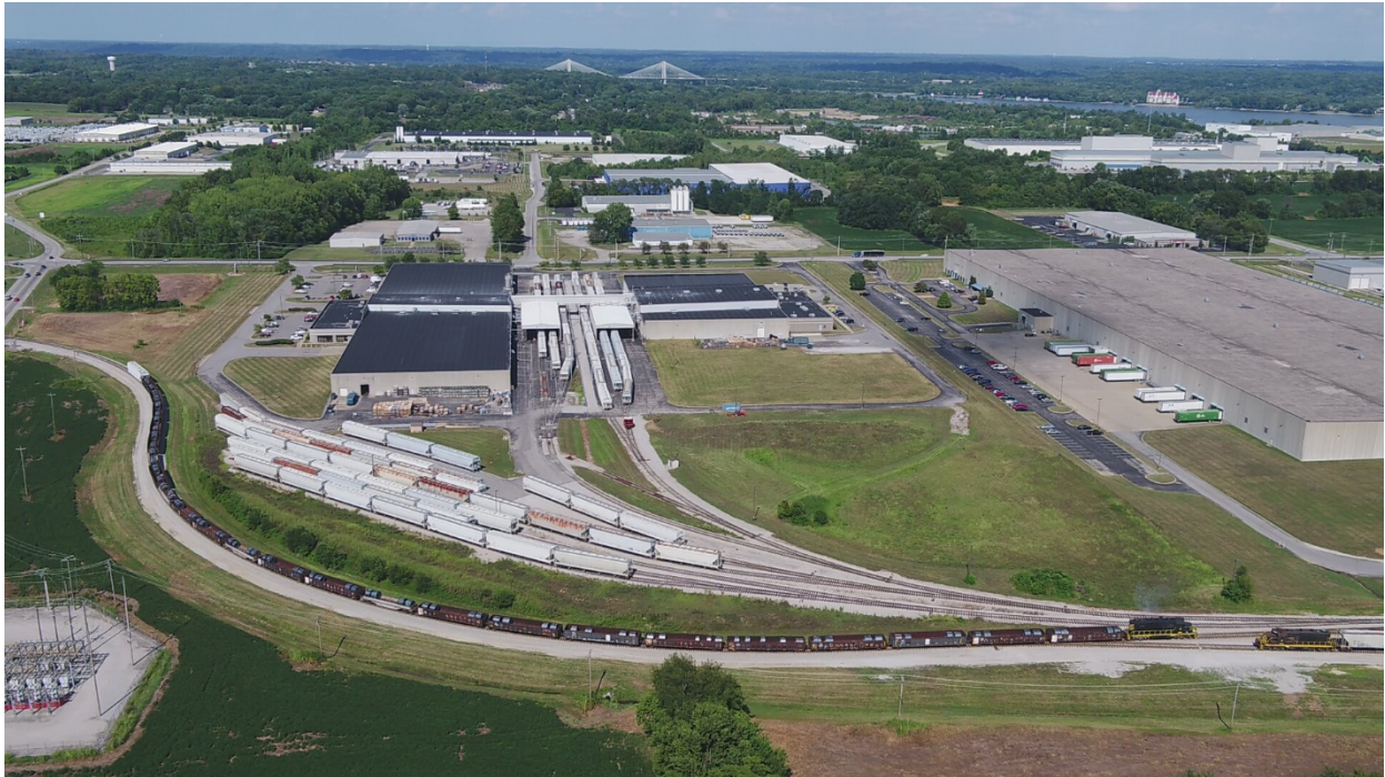
Figure 2-14 – Steel Train Entering Port of Indiana-Jeffersonville in front of Rail-Served Plastics Industries
