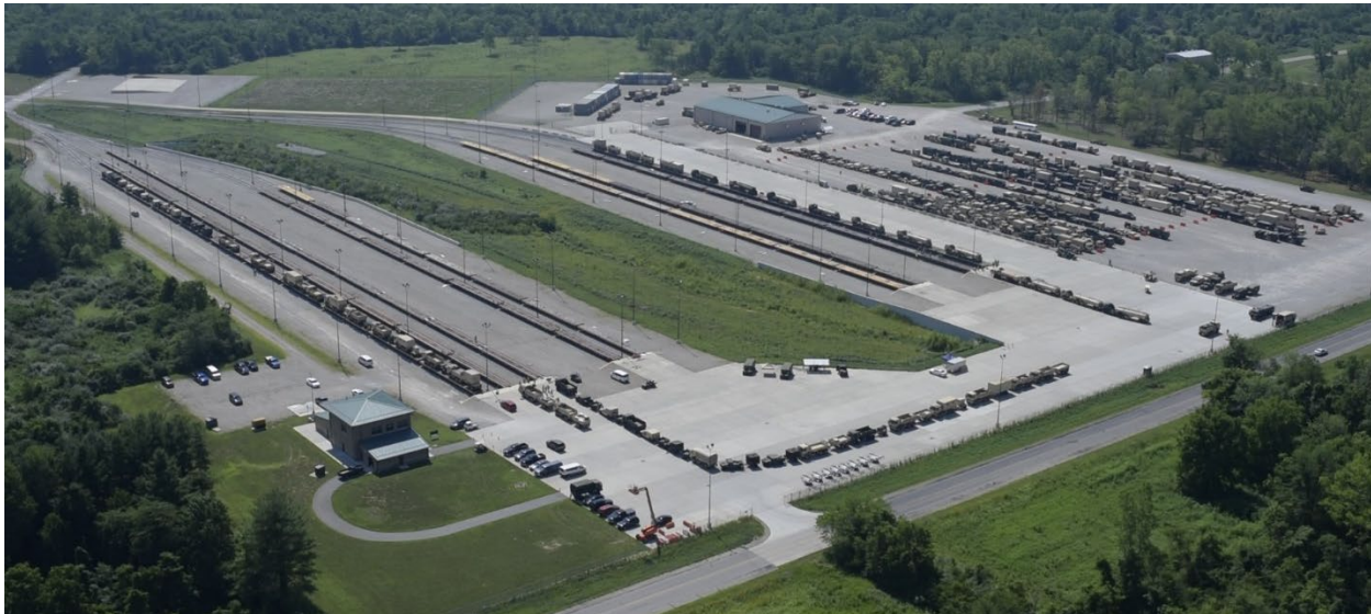
Figure 2-9 – Camp Atterbury Rail Deployment Facility
