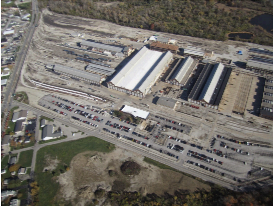
Figure 5-6 – Amtrak’s Beech Grove heavy maintenance facility southeast of Indianapolis
