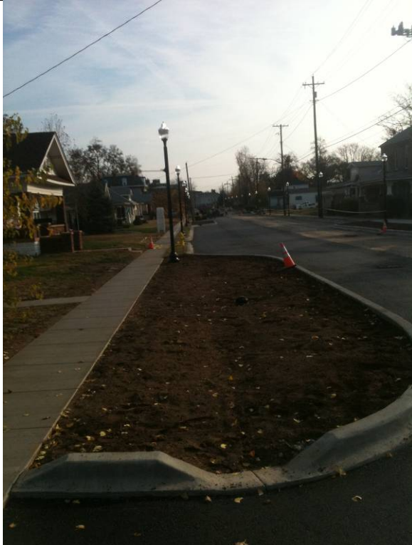
Construction of bioretention bump outs
