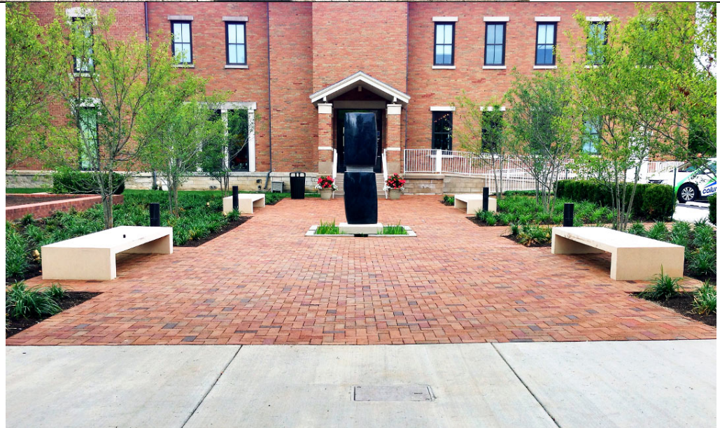
Main plaza after construction with rain gardens
