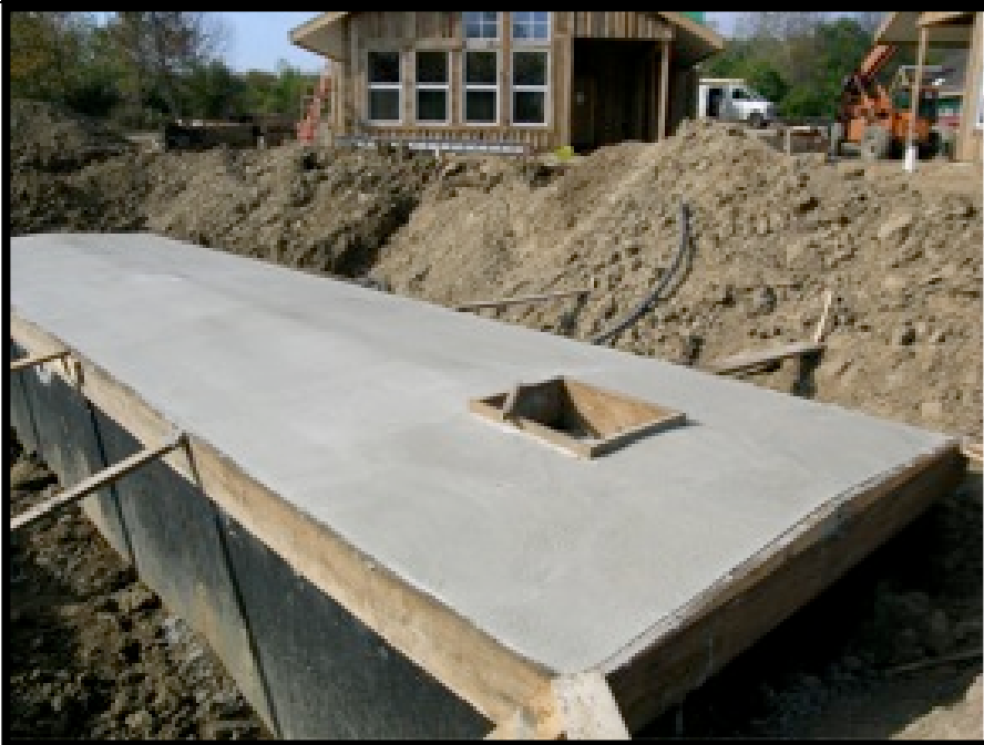
Construction of underground cistern to store rainwater
