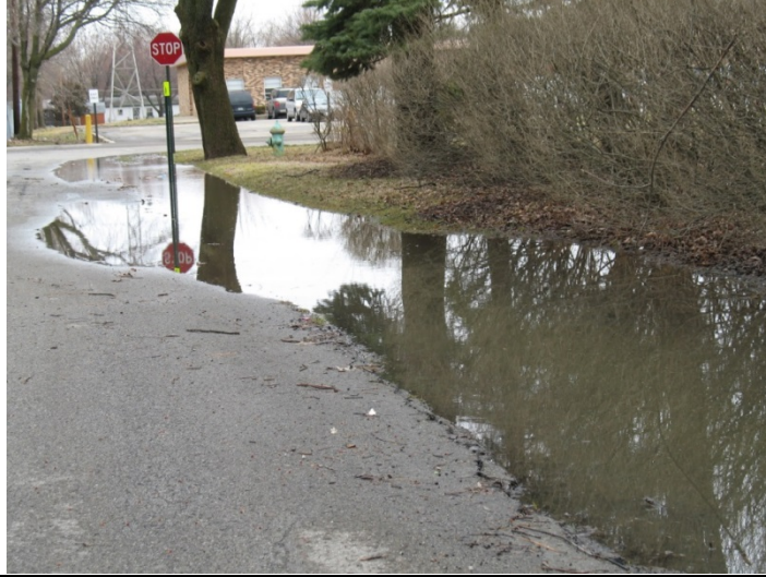
Before photo of typical street flooding
