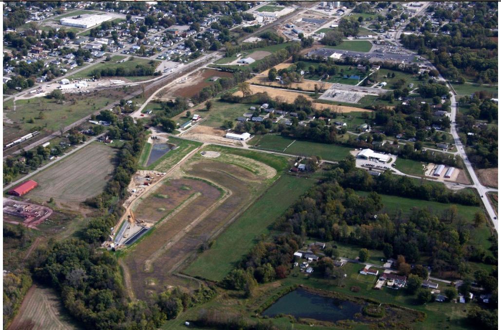
Constructed wetland under construction
