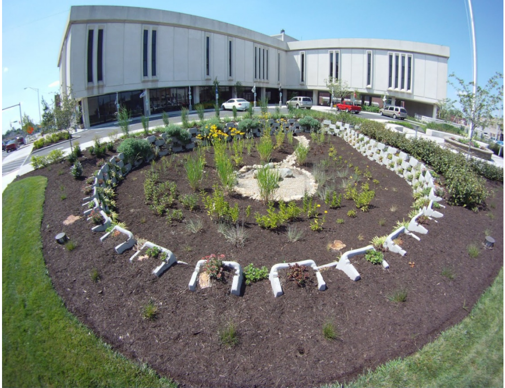
View of bioretention area
