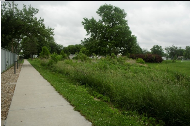
After – East Line showing bioretention area and new sidewalk
