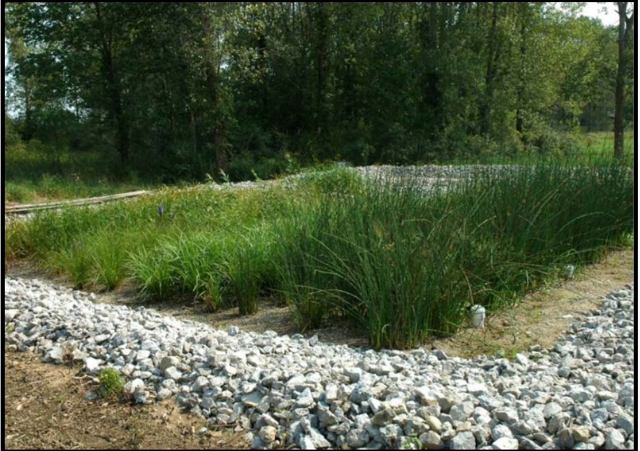
Constructed wetland for effluent treatment
