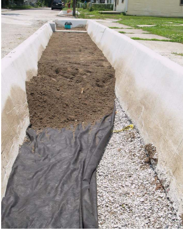
Stormwater Planter under construction
