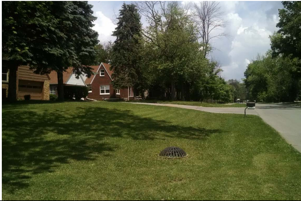
After photo of the hybrid ditch showing the swale and dome grate overflow inlet
