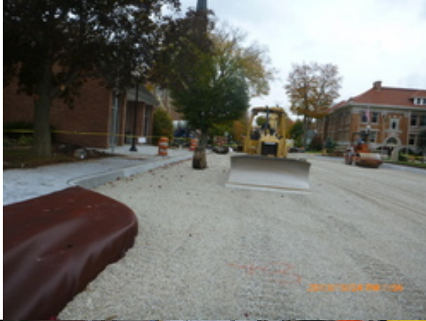
Installation of gravel base
