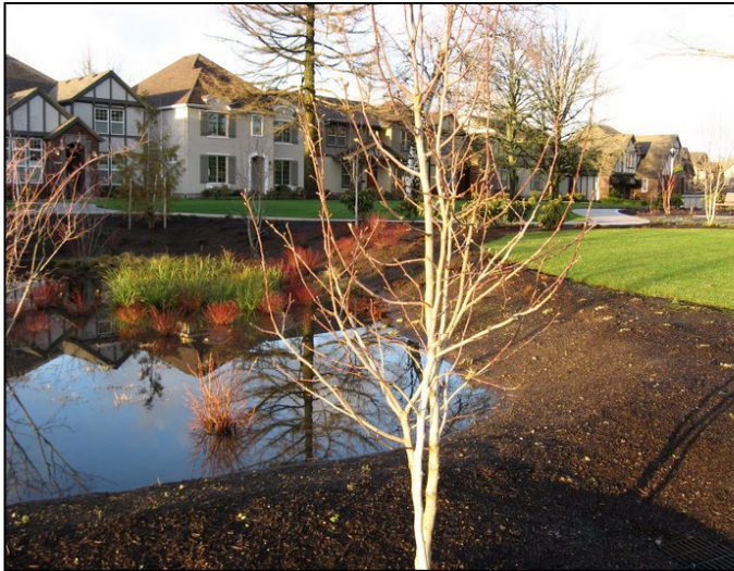
Figure 1 Pond collecting runoff from rooftops, sidewalks, and yards, Wilsonville, Oregon (USEPA, picasaweb)
