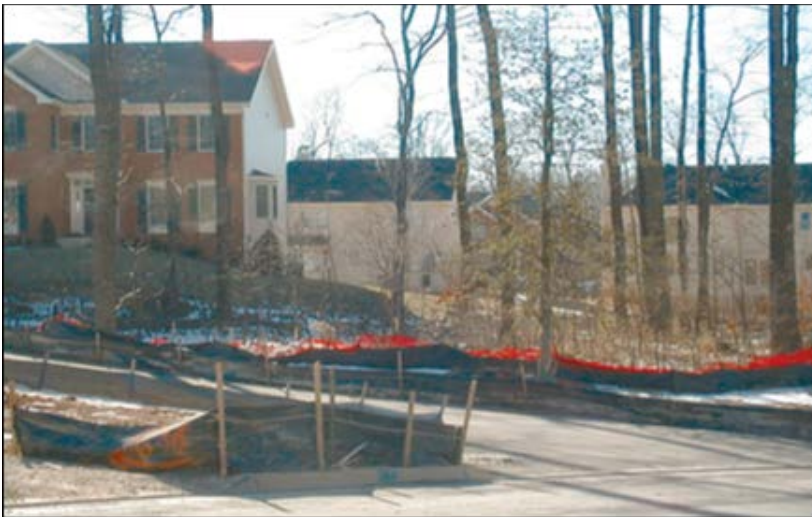
Figure 1 Undisturbed areas are protected during construction (Lake County, OH Stormwater Management Department)
