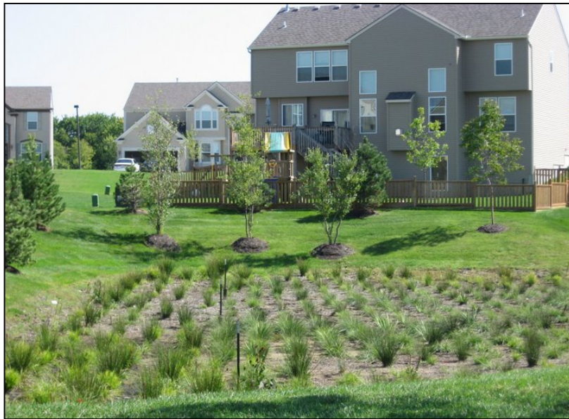
Figure 1 Residential rain garden, Lenexa KS (USEPA, picasaweb)
