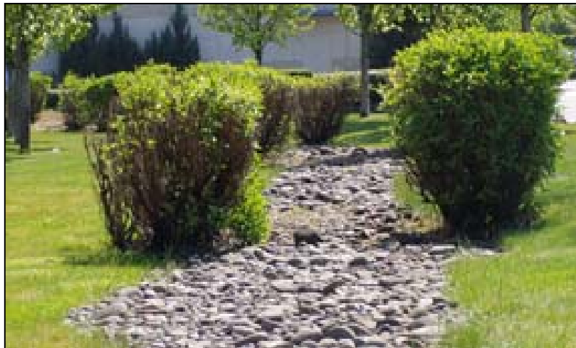
Figure 1 Gravel trench directing water from the parking lot to a vegetated filter strip in Springfield, OR (Springfield Environmental Services Division)
