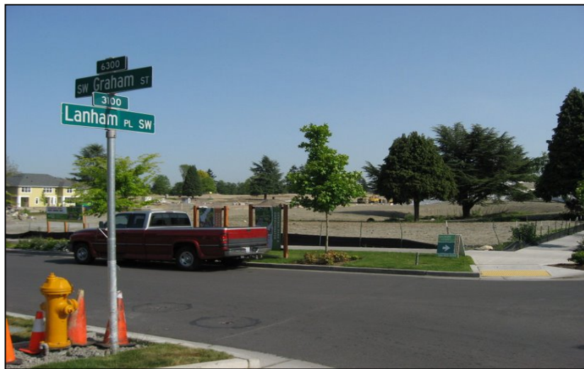
Figure 1 Tree Preservation during construction, Seattle, WA (USEPA, picasaweb)
