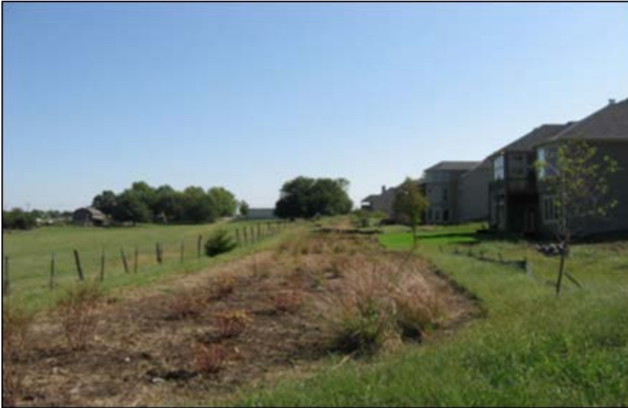
Figure 1 Long swales utilized in areas of natural drainage pathways, Lenexa, KS (USEPA, picasaweb)
