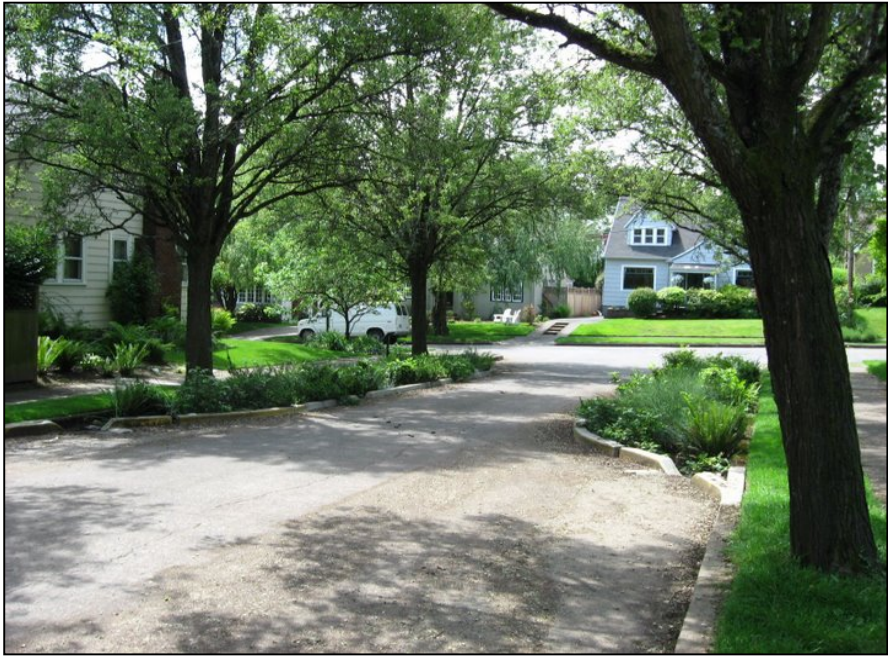
Figure 1 Curb cuts and vegetated areas along a Portland, OR street (USEPA, picasaweb)
